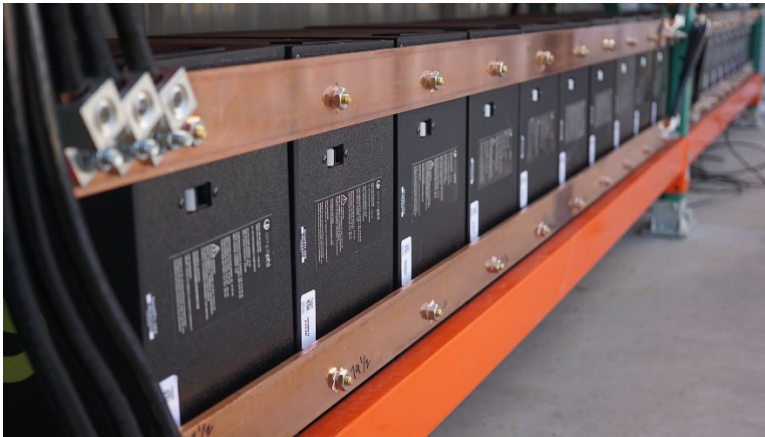
Figure 4.0 – Three PHI Batteries Paralleled Using Direct Bussing
